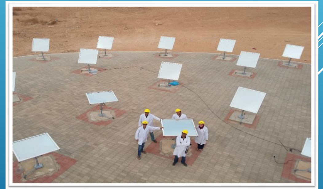
After the completion of 17 heliostats of the construction (2021)
